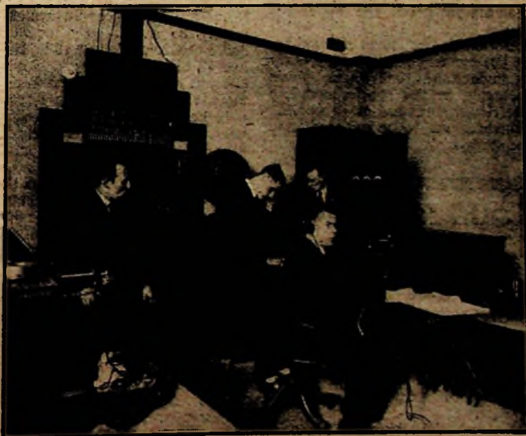
Engineers in the modulating room at 5IT's new studio.
