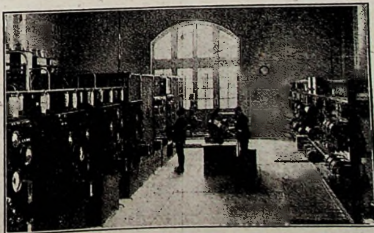
The valve room at Rugby, showing the power units, control tables and switchboard.
